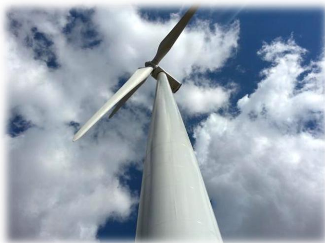
First Salkhit wind turbine
